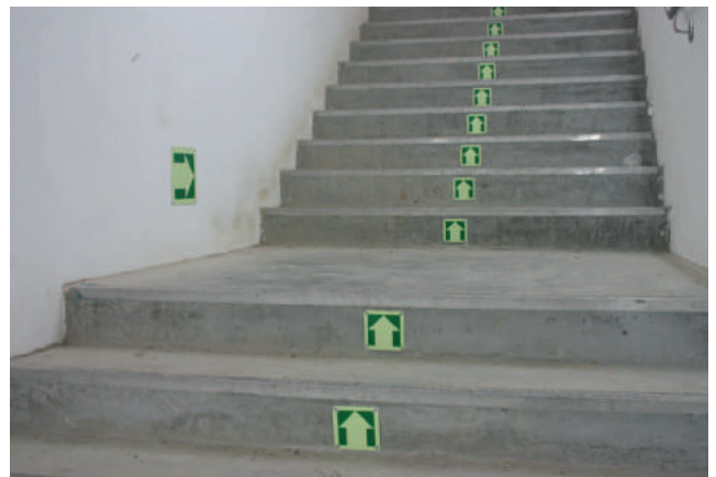
Marine Coastal Expressway - Singapore
